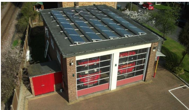
Figure 12 – Solar panels at Frinton Fire Station.
