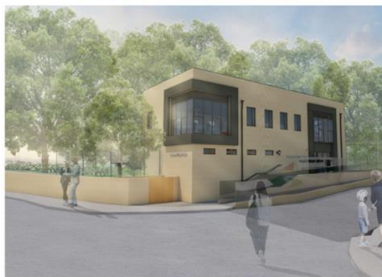
View looking east along Frinton Road
