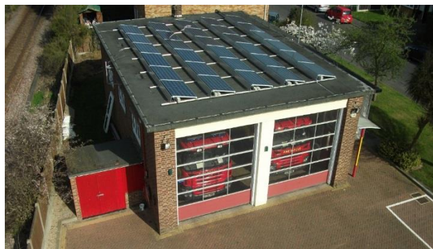
Figure 12 – Solar panels at Frinton Fire Station.
