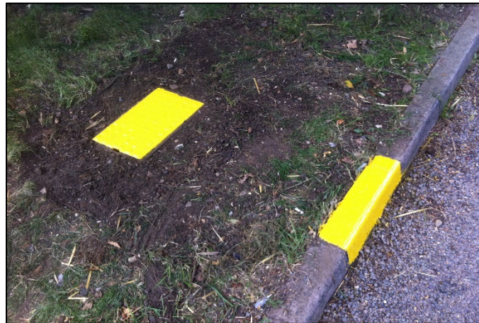
Frame & cover levelled with verge line
