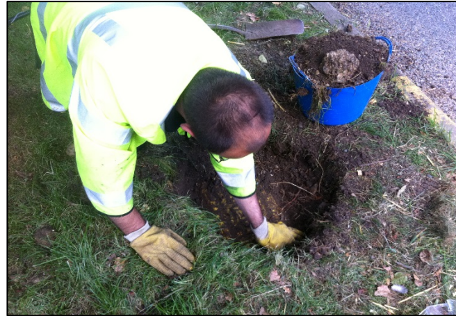
Located with metal detector then excavated
