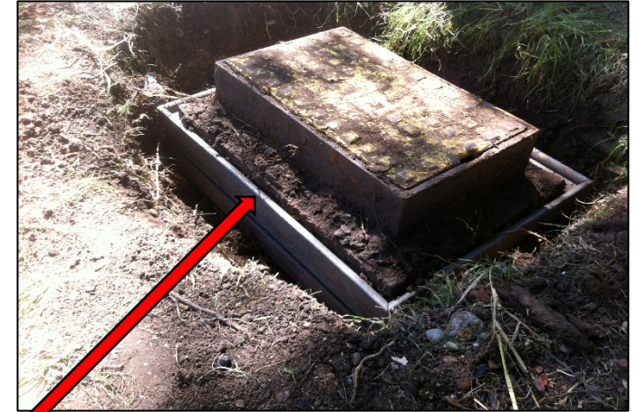
Pit sections installed to raise frame & cover
