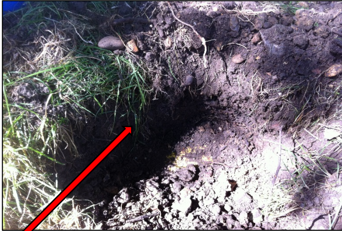
Fire hydrant found unusable - Buried
