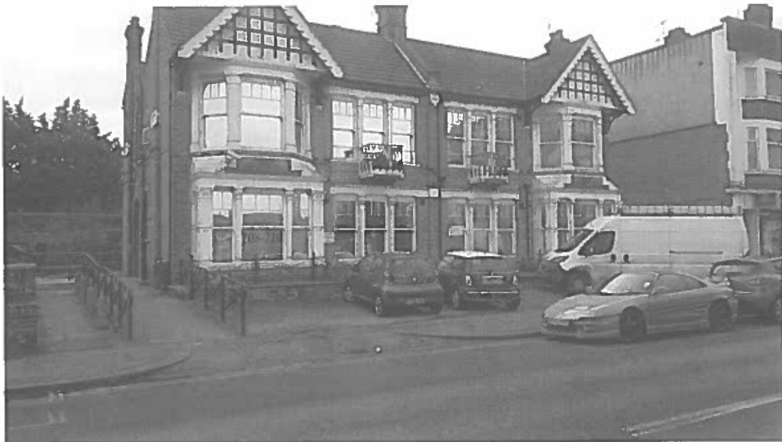
Figure 6 -208 – 210 Southchurch Road – Mixed Use - 5 larger Flats + 11 Rooms
