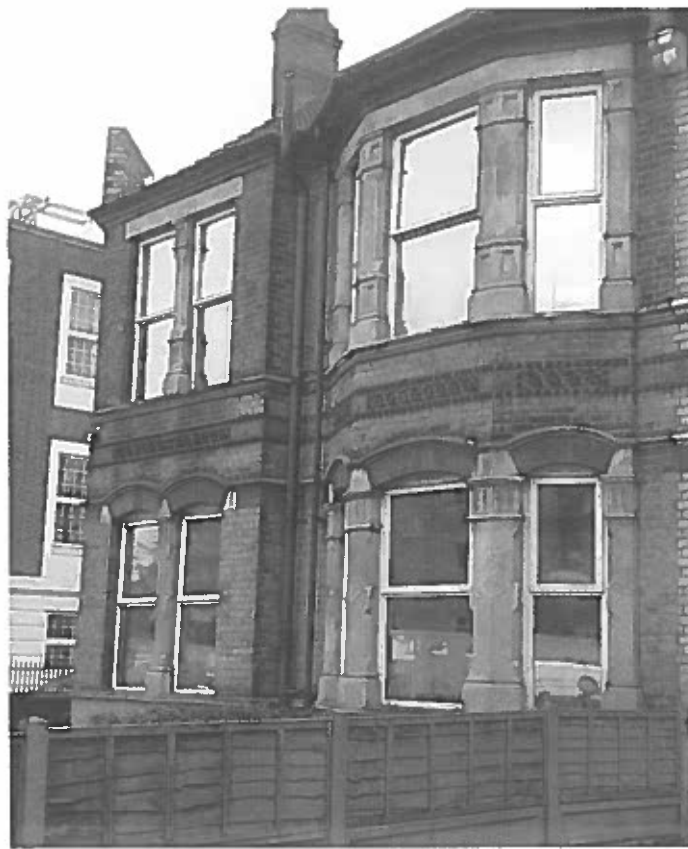
Figure 9 - 228 Southchurch Road – High Risk Unit – 8 Flats
