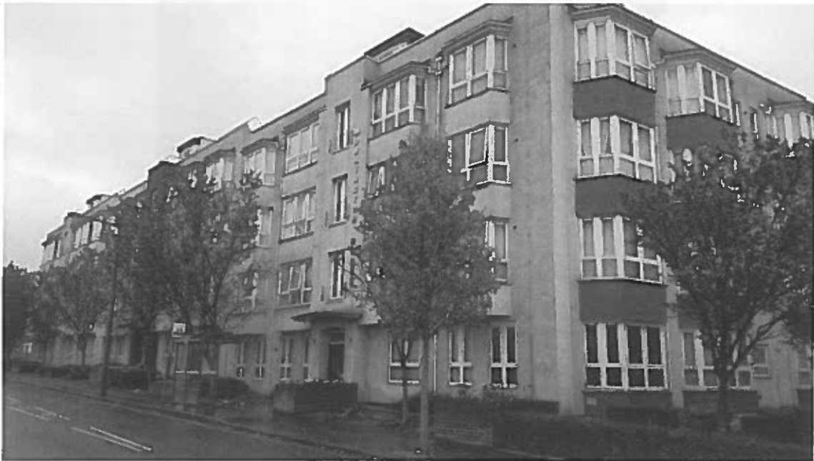
Figure 3 - Mornington House, Southend
